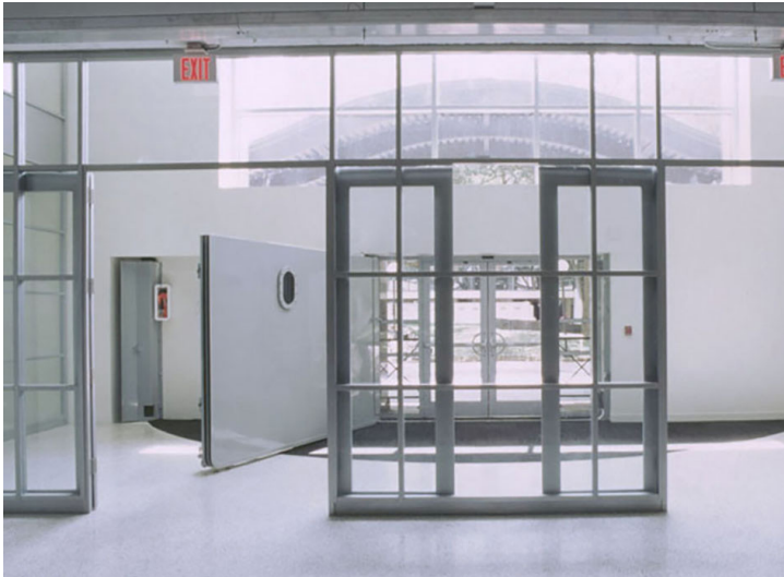
Images: Examples of flood doors installed to protect facilities from flooding conditions.
