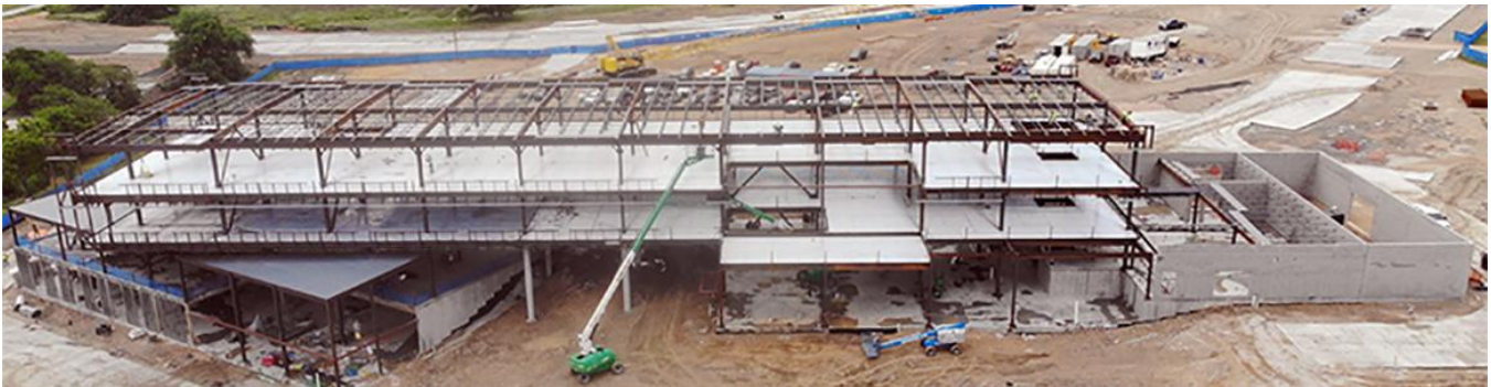
Structural steel installation at Collin College's new Celina Campus.
